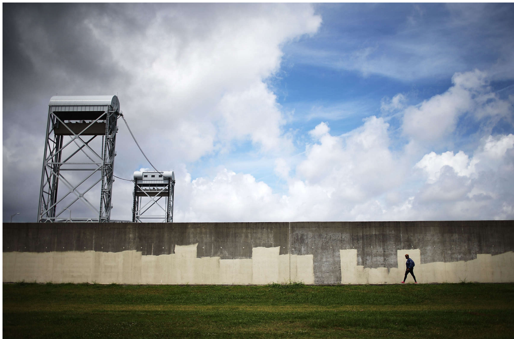
A person walks along the rebuilt Industrial Canal levee wall in the Lower Ninth Ward on May 18, 2015, in New Orleans, Louisiana.
